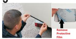
Add Tape: Use the pre Cut sure seal tape in Kit bag "D". Peal off the back of the tape to gain access to the adhesive back. Cut the tape to the length of the hinge and transom bracket.
