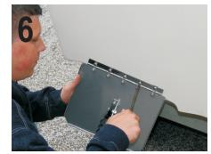
Attach the Plate: Using a philip head screw diver attached the plate using the #14x3/4 sheet metal screws that came in bag "A". Do not overtighted these and don't use a screw gun.
